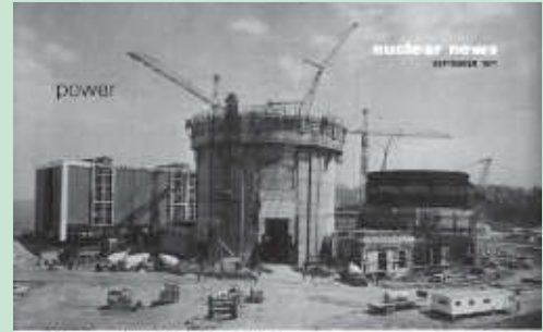
Calvert Cliffs, construction site, September 1971
