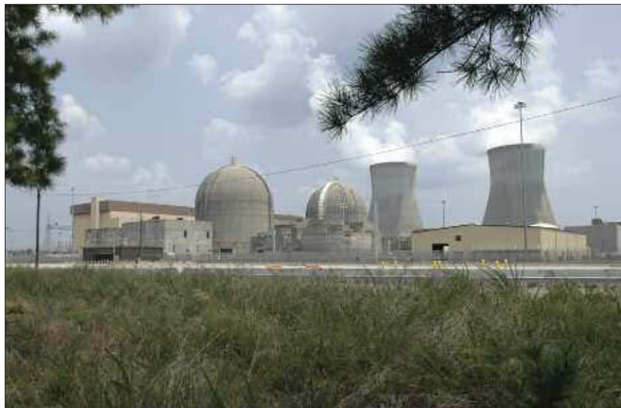
Vogtle: Operating licenses for both units renewed in June by NRC
