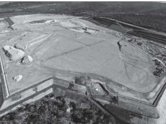
The ITER construction site
