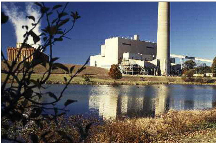
Hatch: Elevated levels of tritium detected on the plant's property, not off site
