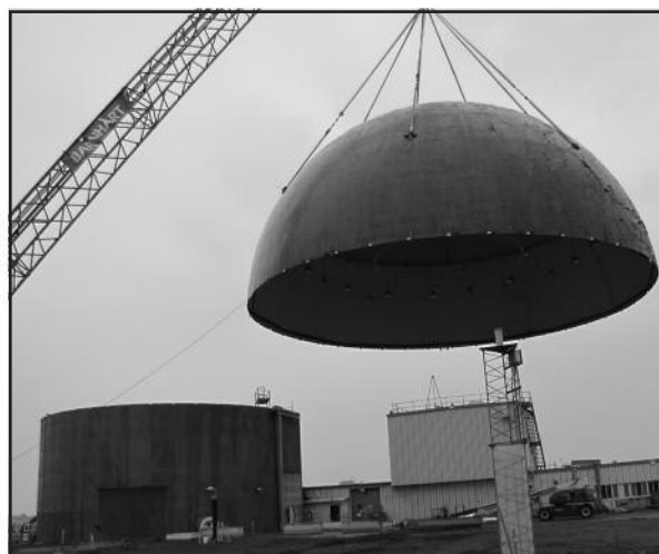
REACTOR DOME REMOTELY CUT
