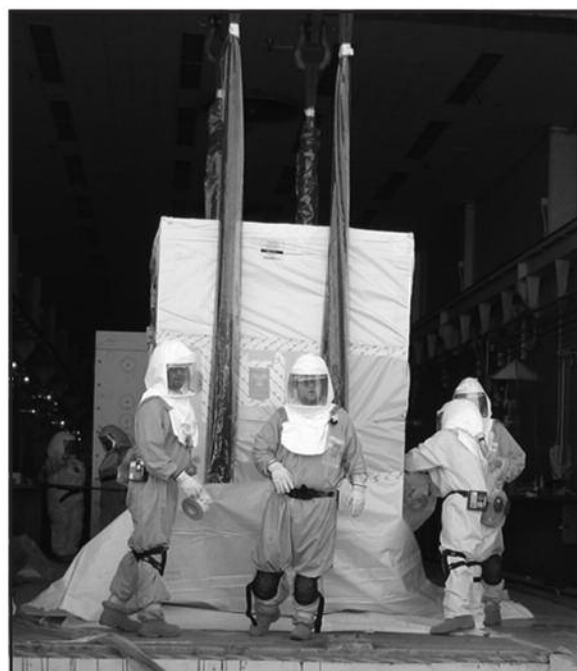
HOT CELLS WIRE SAWED FLUSH TO FLOOR
