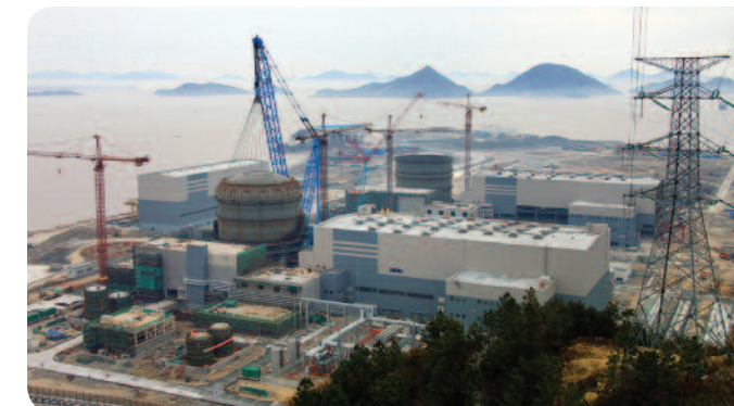
Sanmen Units 1 and 2, China
