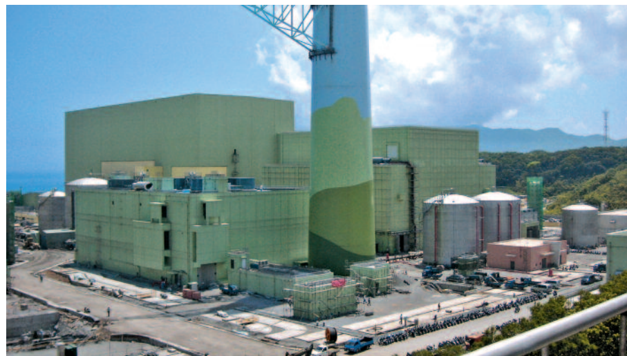
The Lungmen facility features Advanced Boiling Water Reactor technology, and when both units are completed, will be rated at 2,700 megawatts.
