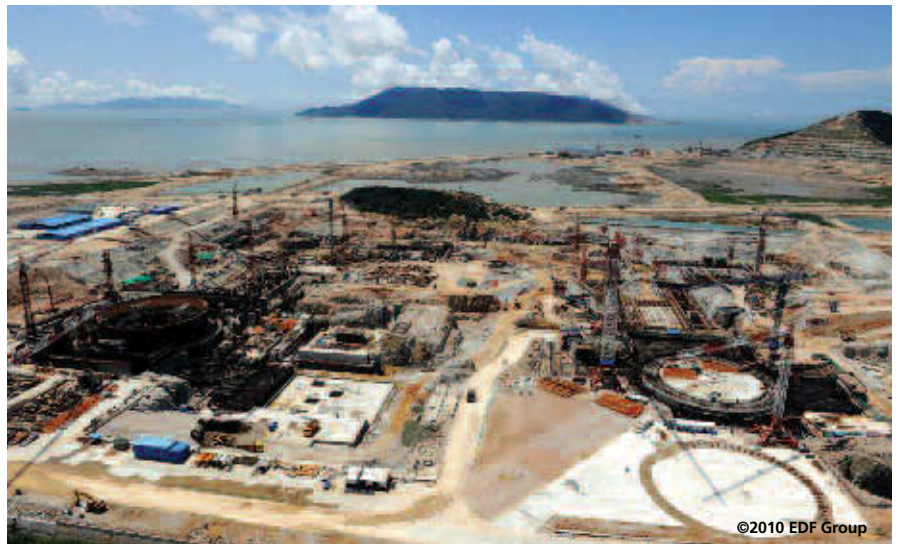
Taishan Units 1 and 2 now under construction in China.
