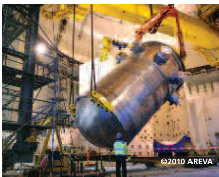
Installation of reactor pressure vessel at Olkiluoto, Finland in June 2010.
