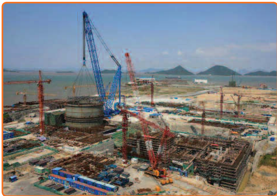
Containment Vessel 2nd Ring placement at Sanmen Unit 1, China
