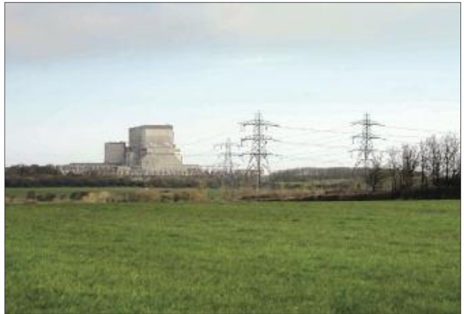
British Energy's Hinkley Point B (Photos: British Energy)
