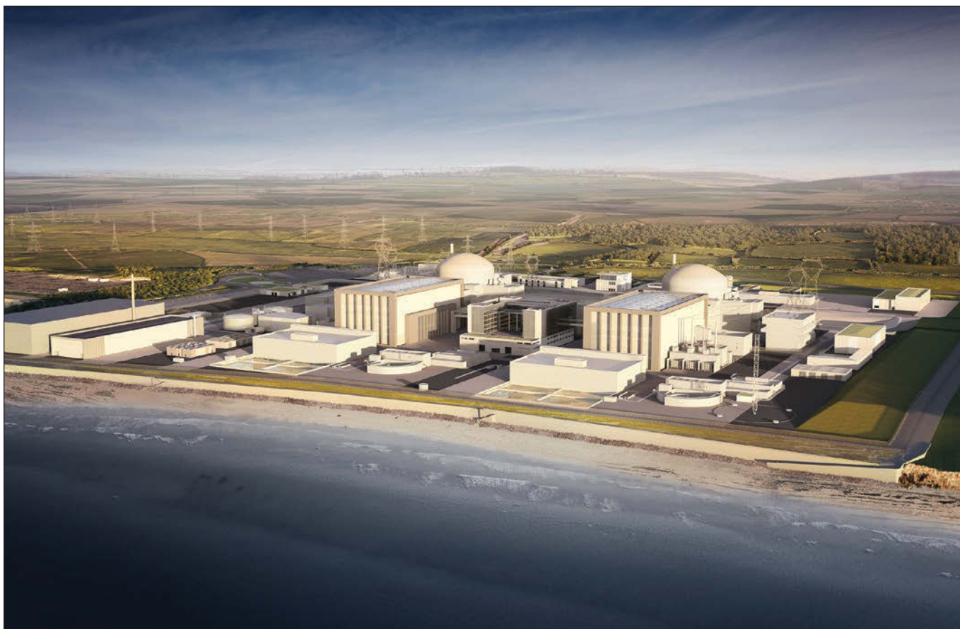
A computer-generated image of the Hinkley Point C plant, which will consist of two 1,600-MWe UK EPRs.
