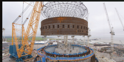
"Big Carl", the world's largest land-based crane, lifts the final liner into place at Hinkley Point C.
