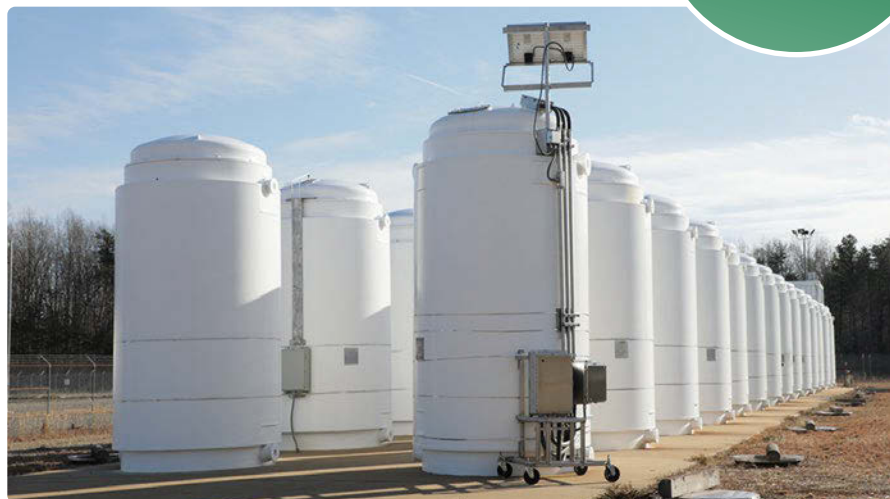
The high-burnup research cask (center) stands with other spent nuclear fuel dry storage casks at the North Anna ISFSI in Virginia. (Photo: Dominion Energy)
