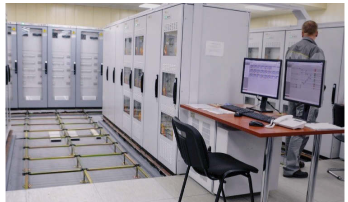
Digital safety systems require fewer equipment racks, reducing the total data center footprint.
